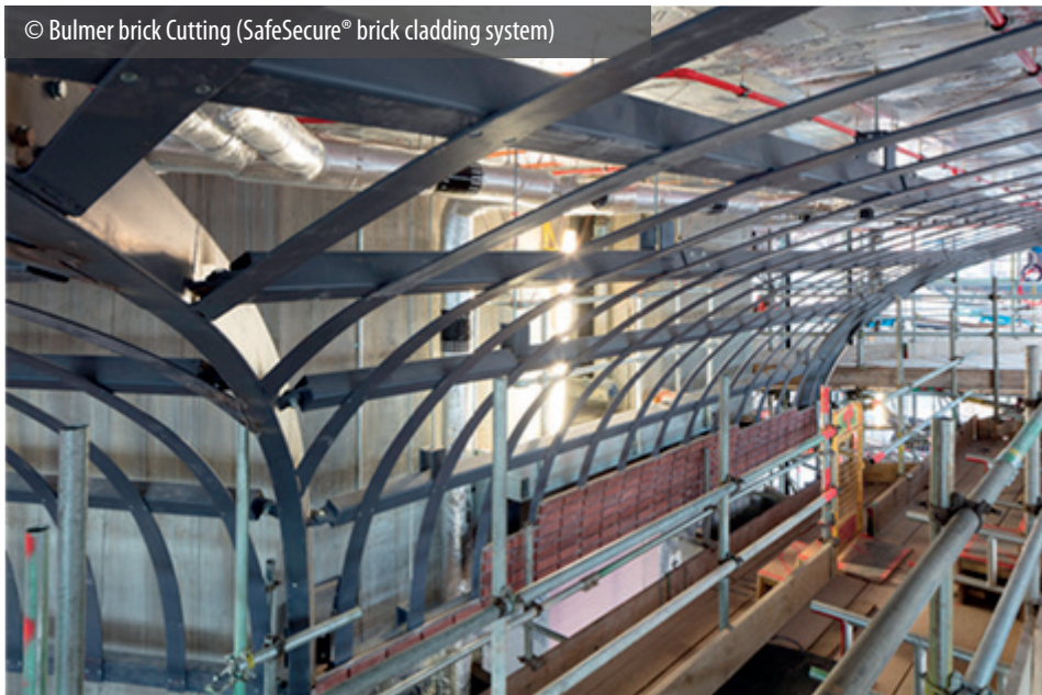
© Bulmer brick Cutting (SafeSecure® brick cladding system)
